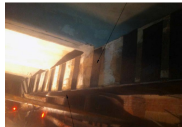
Fig. 9. Reinforcement of floor beams
