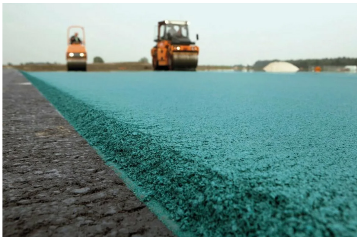
Fig. 3. Testing of asphalt concrete mix using rubber crumbs
