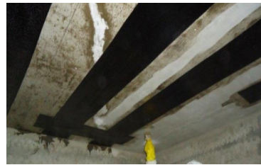
Fig. 7. Reinforcement of floor slab
