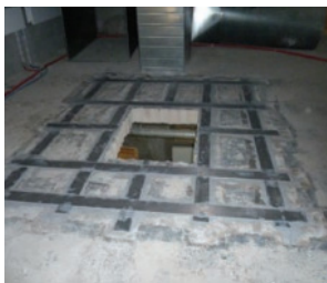
Fig. 8. Reinforcement of the floor opening
