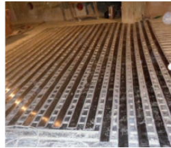
Fig. 5. Reinforcement of foundation slab
